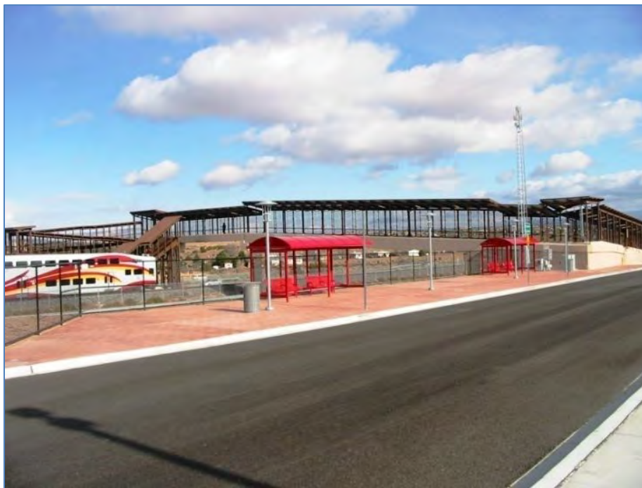
Rail Runner Station at NM 599
