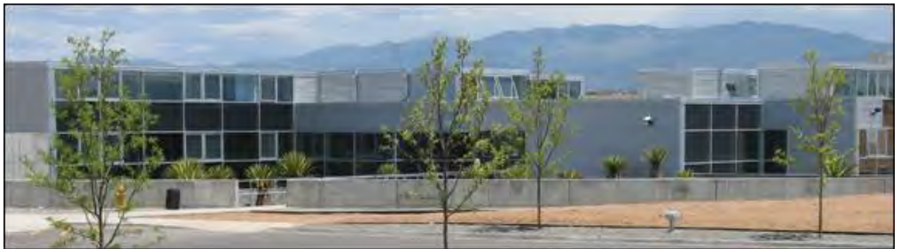
Santa Fe County Public Works Complex, Santa Fe, NM
