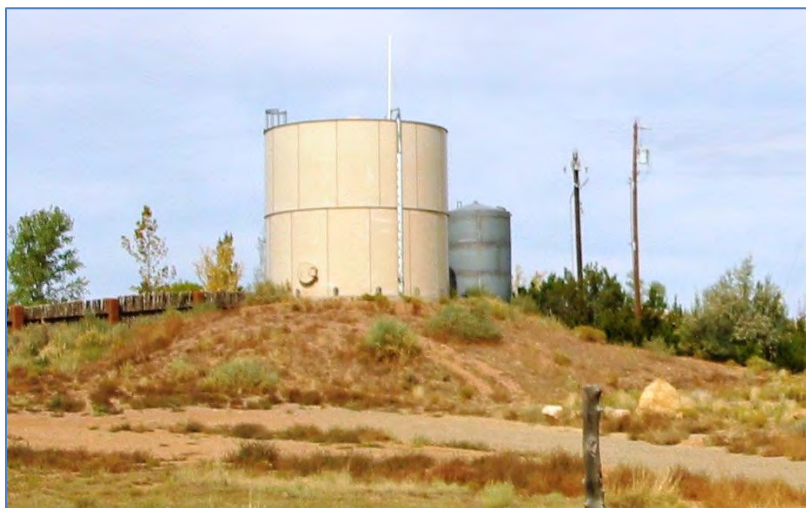
Galisteo Water Tank
