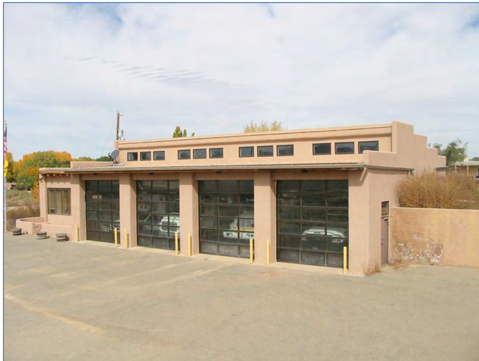
Galisteo Fire Station
